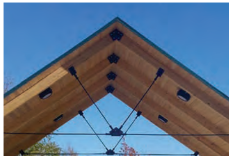
Rod and clevis ties
