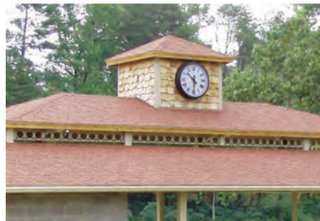
Clock on enclosed custom cupola
