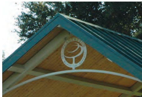
Curved tie beam with laser-cut medallion
