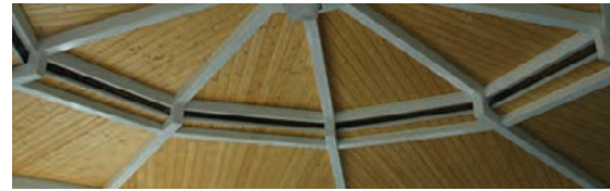
Interior view of Vented roof option
